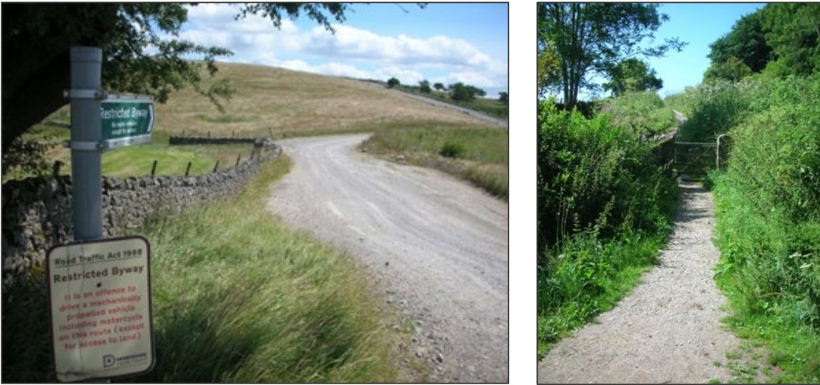
Figure 4: Examples of made unsealed surfaces on a road (left) and a path (right).
