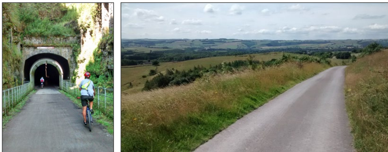
Figure 3: Two examples of made sealed surfaces on roads.
