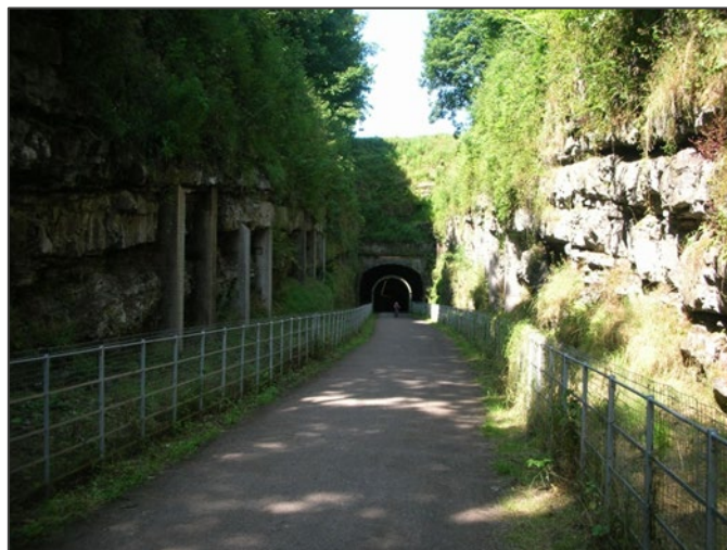
Figure 7: This route passes through a specially built construction underneath the normal terrain surface.
