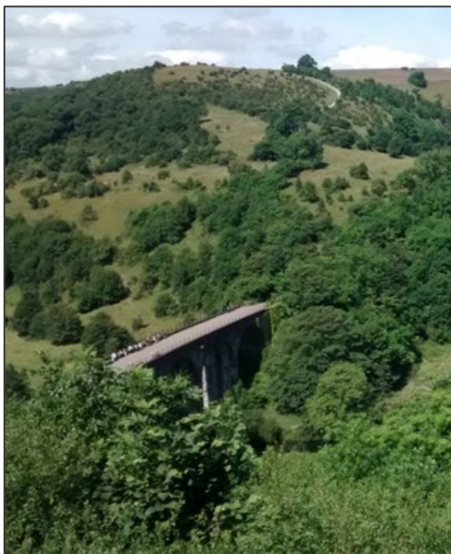
Figure 6: Example where a RouteLink is supported or suspended above ground level on a manmade structure.
