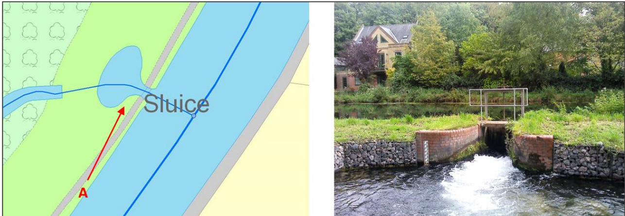
Figure 9: An example of a watercourseInteraction which could be modelled through point referencing.
