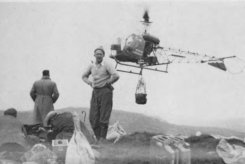
Coming in with a load; pillar construction in progress (Wester Ross)
