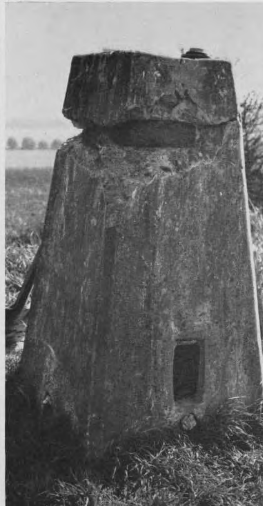
Wilford Brickworks (tertiary) near Nottingham; an unsuccessful attempt to remove the tribrach
