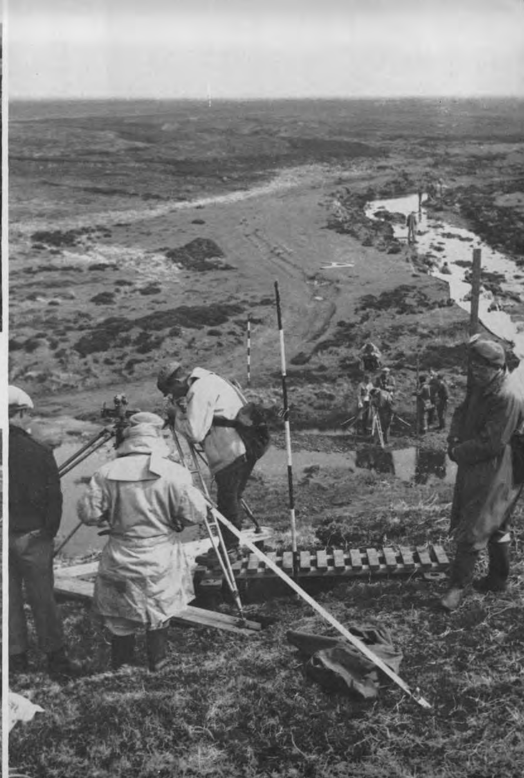
Crossing the Burn of Lyth just north of Hillhead Farm. 'A' frame in use
