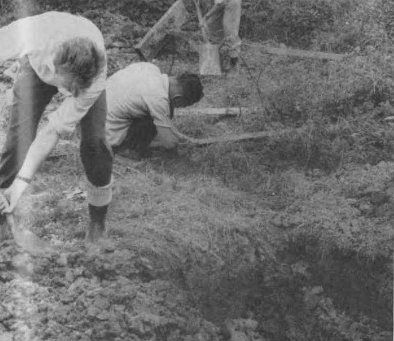
Excavating for footings
