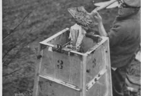
Filling the shuttering
