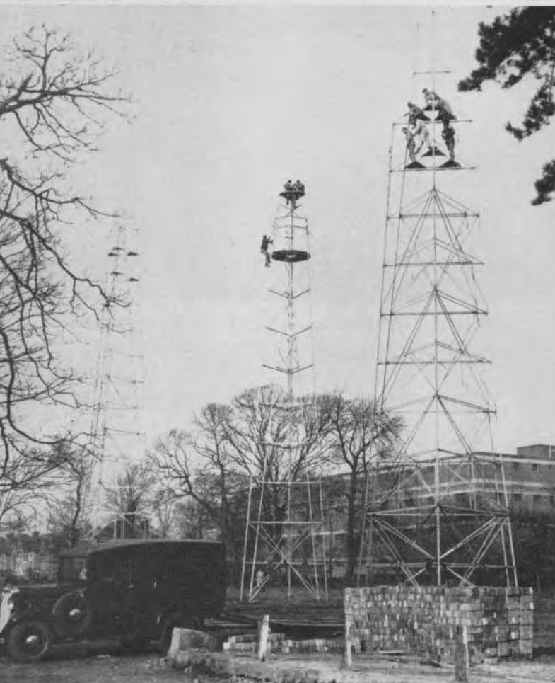
Practising tower erection, Southampton
